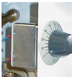
Typical View of Cooling Lock Thermostat
